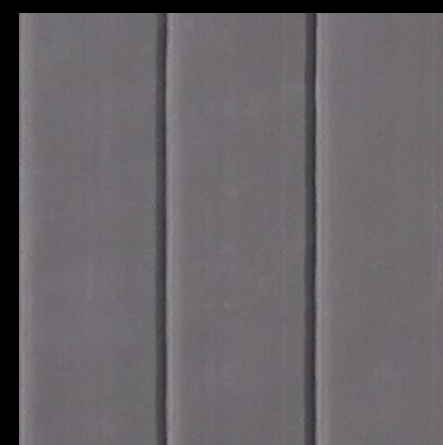
Standing Seam Metal Cladding
